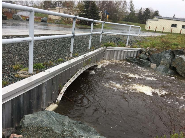
Figure 8: Existing Capacity Issues - Arch Bottomless Culvert Mahon's Lane
