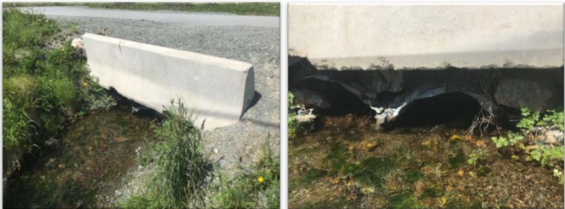
Figure 13: Existing Culverts In Poor Condition - Compressed by Jersey Barrier
