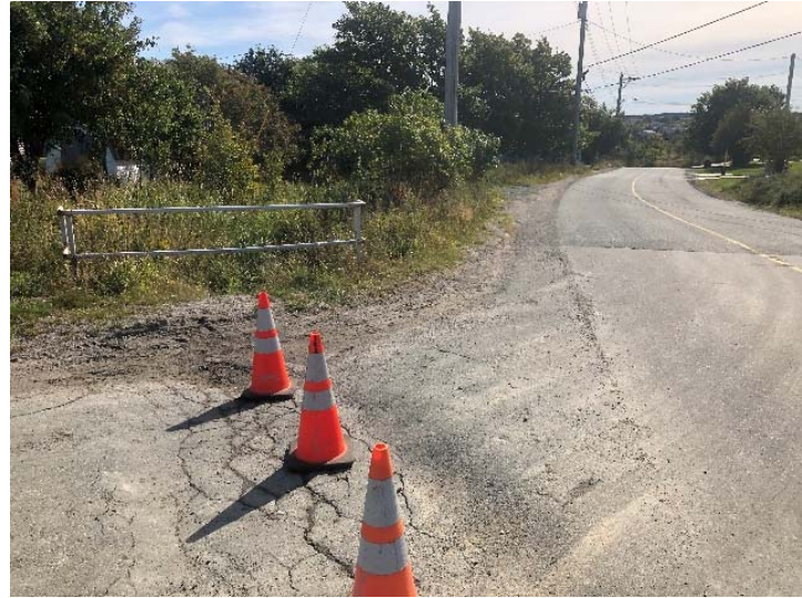
Figure 14: Partially Collapsed Section of Storm Pipe - Country Drive/Hickey's Lane
