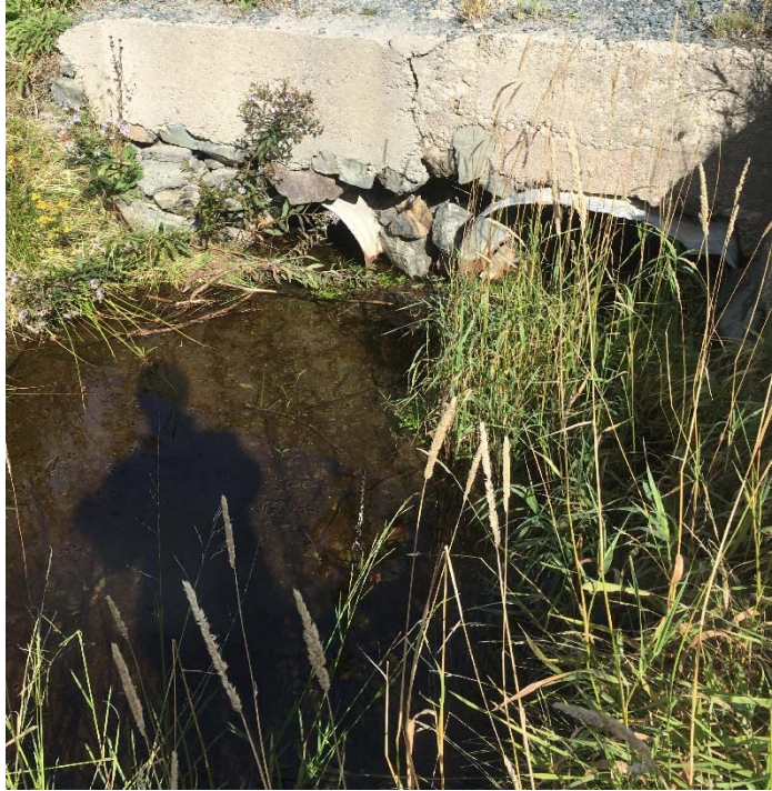
Figure 9: Culverts Crossing Quigley's Lane in Poor Condition
