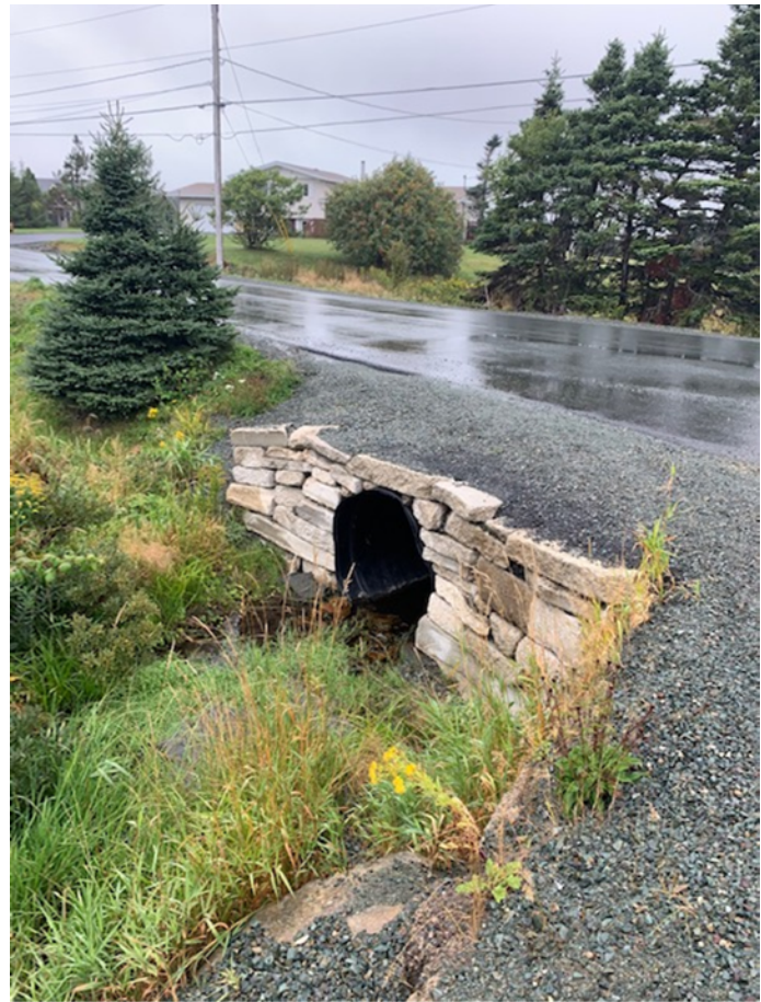
Figure 10: New 1200mm HDPE Pipe - Quigley's Lane
